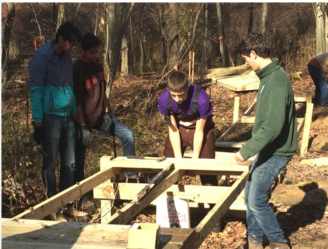
Leveling a section and securing to the upright posts.
