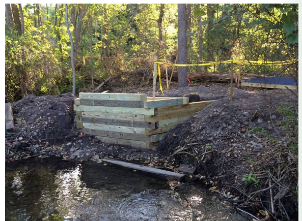
This is what a foundation looks like.
