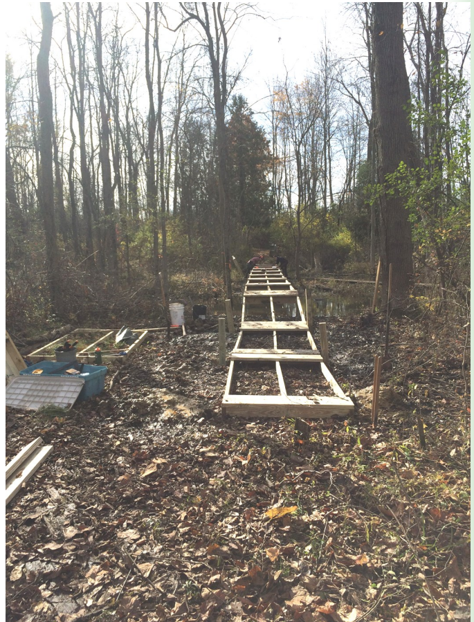
Laying out the sections to align with the Beaver Bridge.
